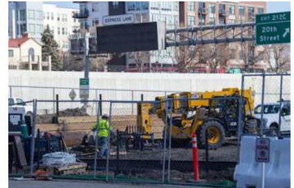
KATHLEEN LAVINE, DENVER BUSINESS JOURNAL Construction at 1701 Platte St.
